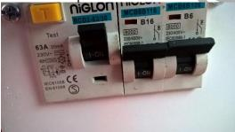
A 16amp Circuit breaker is provided for short circuit protection.
